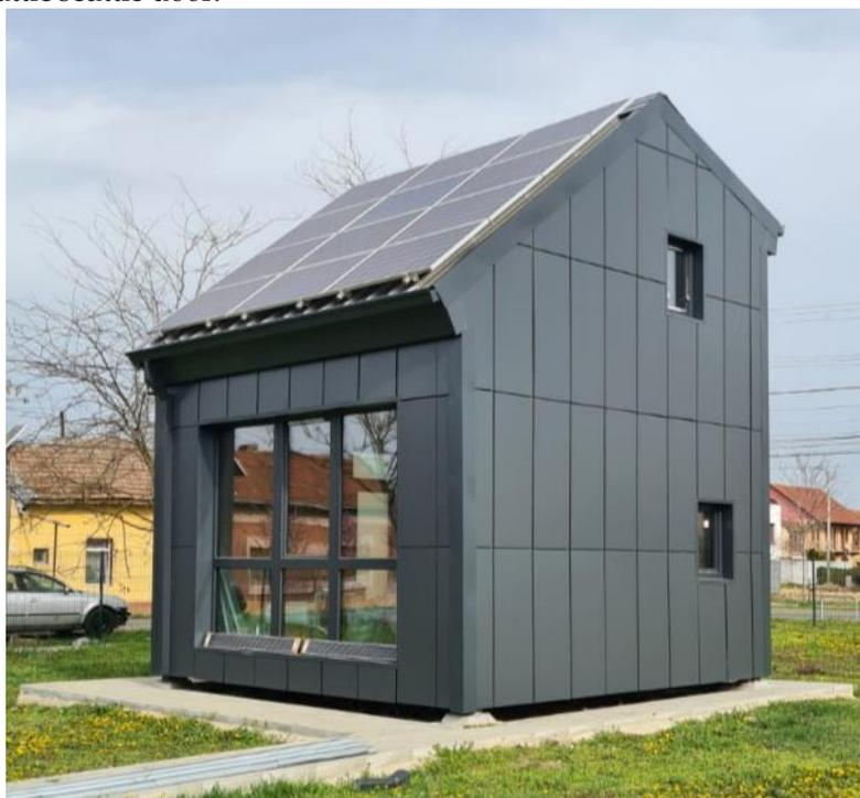
**Figure 9.** LSF experimental module.
