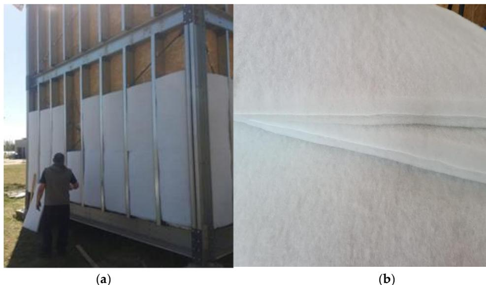
**Figure 12.** Recycled-PET thermal wadding: (a) Installation phase at the construction site; (b) Layers of insulation before installation.
